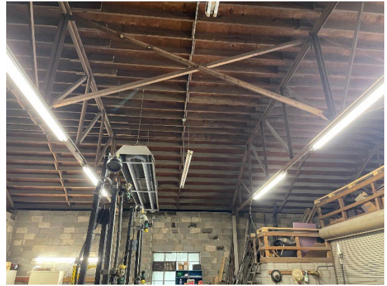
Photo 14 – Steel Truss bracing
