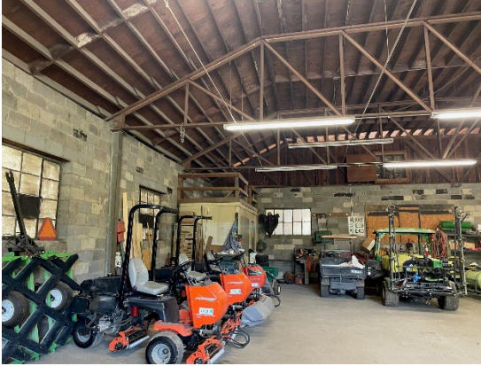
Photo 13 – Steel Truss with wood purlins
