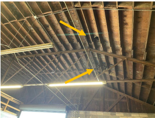
Photo 17 – Water Damage to Plywood
