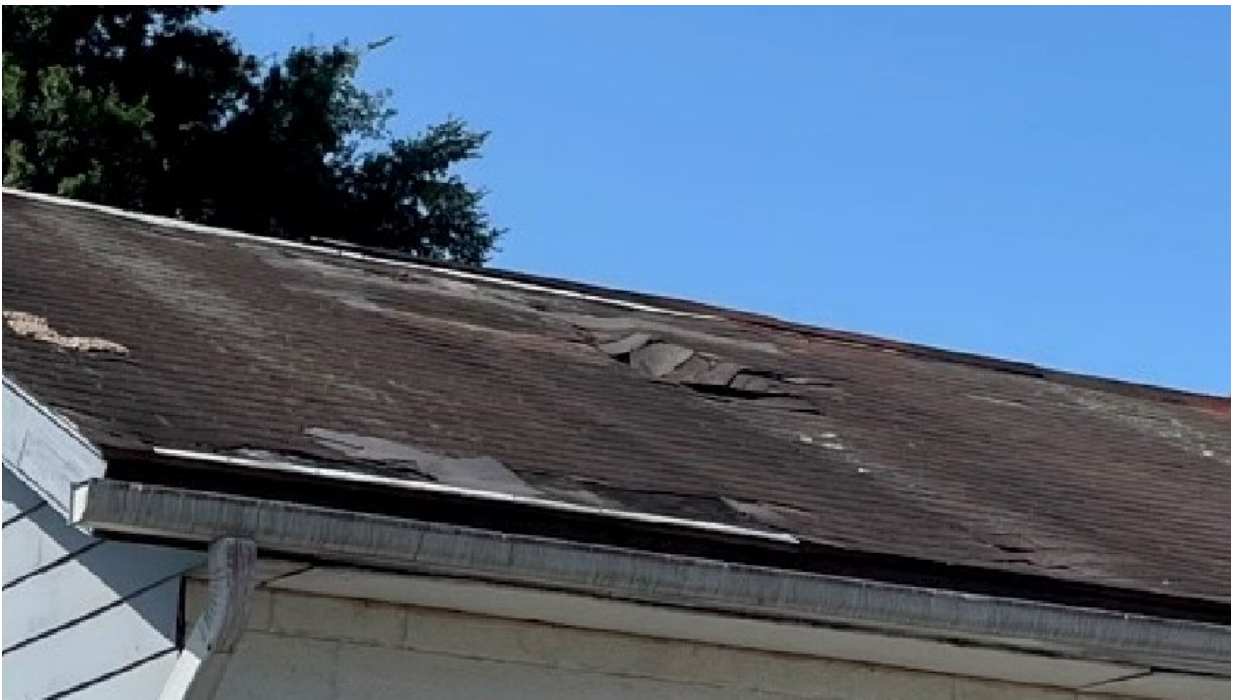
Photo 21 – Shingle Roof has Exceeded Life
