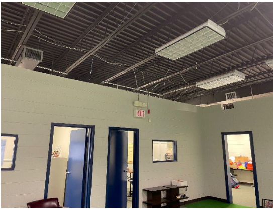
Photo 5 – Steel Bar Joists
