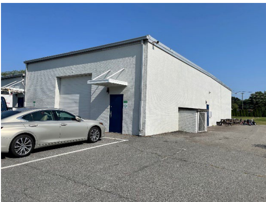
Photo 9 – Exterior Load bearing CMU
