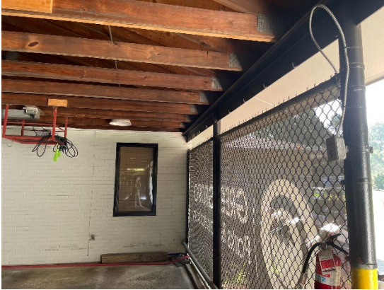
Photo 3 – Wood Roof Trusses & Perimeter Steel Beams
