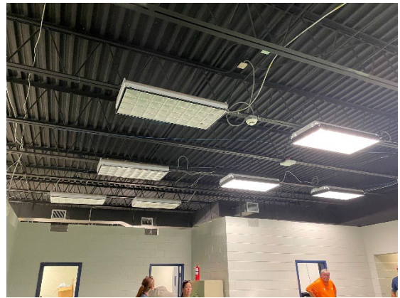
Photo 6 – Steel Bar Joists
