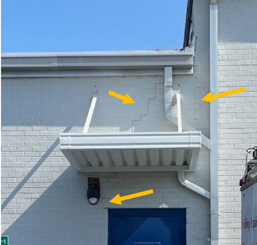
Photo 11 – Observed Exterior Crack
