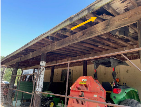
Photo 24 – Water Damage to Plywood
