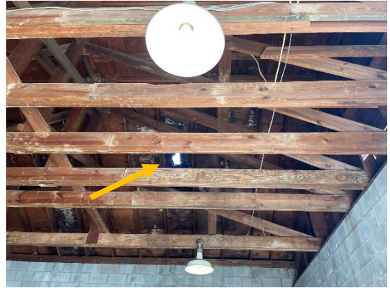
Photo 20 – Light visible thru Water Damage to Plywood
