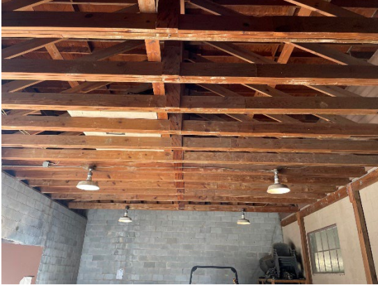
Photo 19 – Wood Roof Trusses
